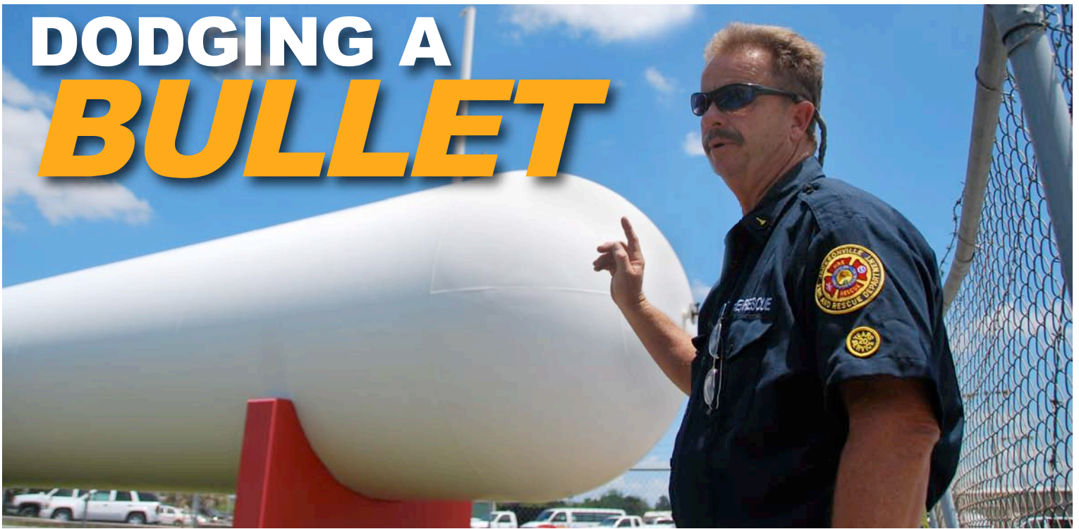
Eng. 7's Lt. Mark Johnson explains how crews mitigated a propane leak in this 30,000 gallon tank on April 7 at Fleet Management.
